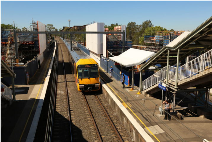
Concord West Station
